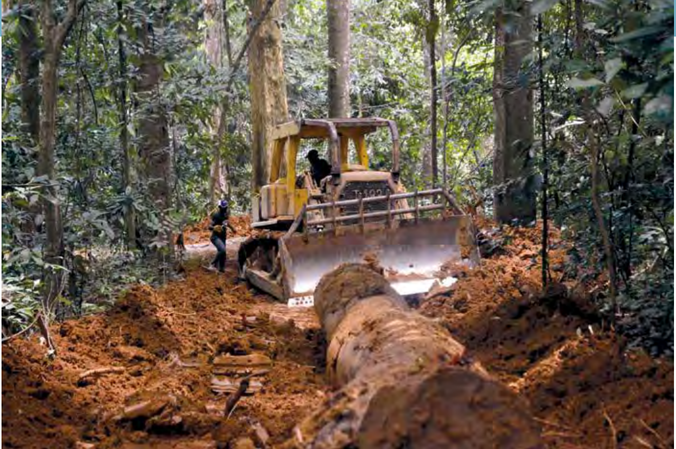
A bulldozer opening a secondary logging road in a forest concession in Gabon. Source: ANPN
